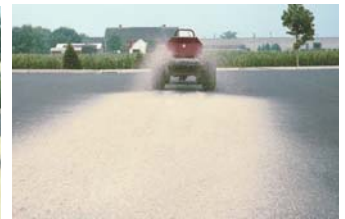
The wet sand was applied uniformly across the blacktop, an amazing feat.
